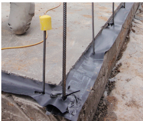
Reinforcement bars and damp proof course installed
