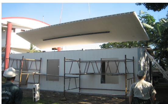
Sequence of photographs showing lifting of roof panel into position with under panel spreader bar
