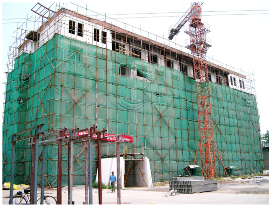
Multi-storey building using tower crane
