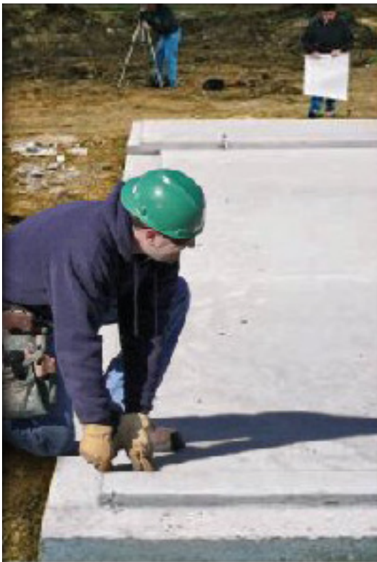
Checking the accuracy of the slab
