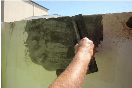
Repair to mid section of crushed panel
