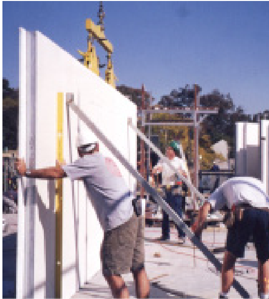
Panel being propped
