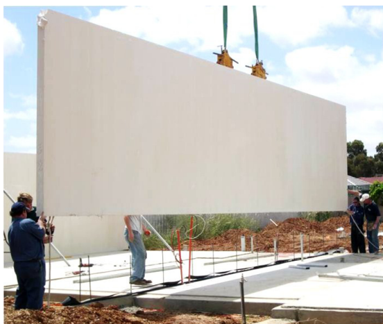
Double lifting jaw lift of large panel
