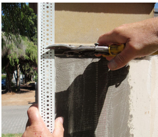
Cutting external corner bead to size
