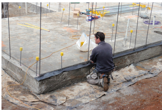
Prepare slab for panel installation
