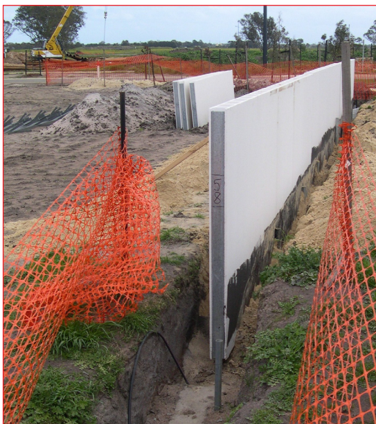
Rapidwall fence preparation for filling with sand.
