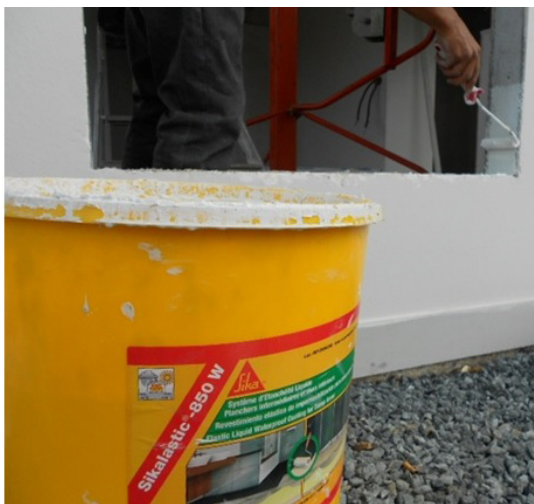
Waterproofing with liquid elastomeric membrane for windows and doors
