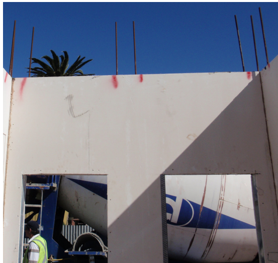
Reinforcement bars inserted ready for upper walls
