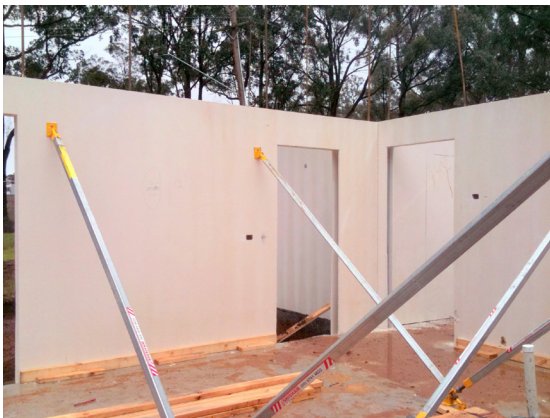
Props in position, note 'whale' boards also installed to assist in positioning panel
