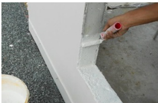
Waterproofing with liquid elastomeric membrane for windows and doors
