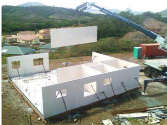
Craning panel into position.
