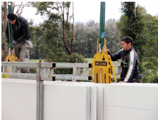
Lifting jaws being lowered into position
