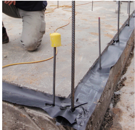
Reinforcement bars and damp proof course installed
