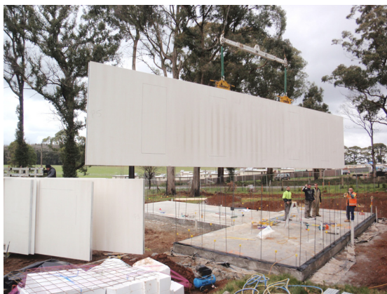
Panel being lifted into position
