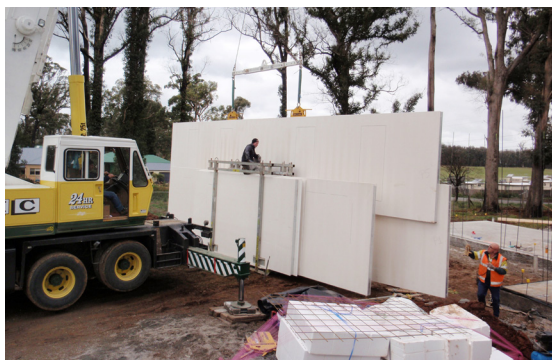
Removing panel from stillage
