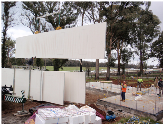
Panel being removed from stillage
