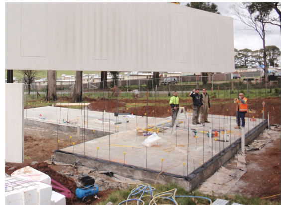
Panel being lifted into position
