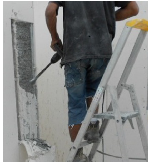
Repairing a concrete blowout
