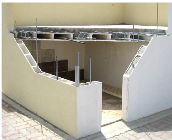
Display section showing Rapidfloor construction
