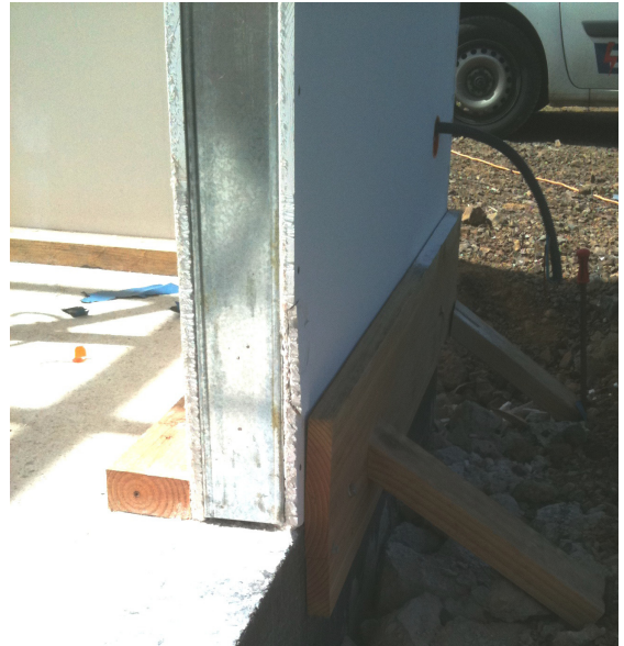
Whale boards positioned to assist panel placement with external concrete fill supports
